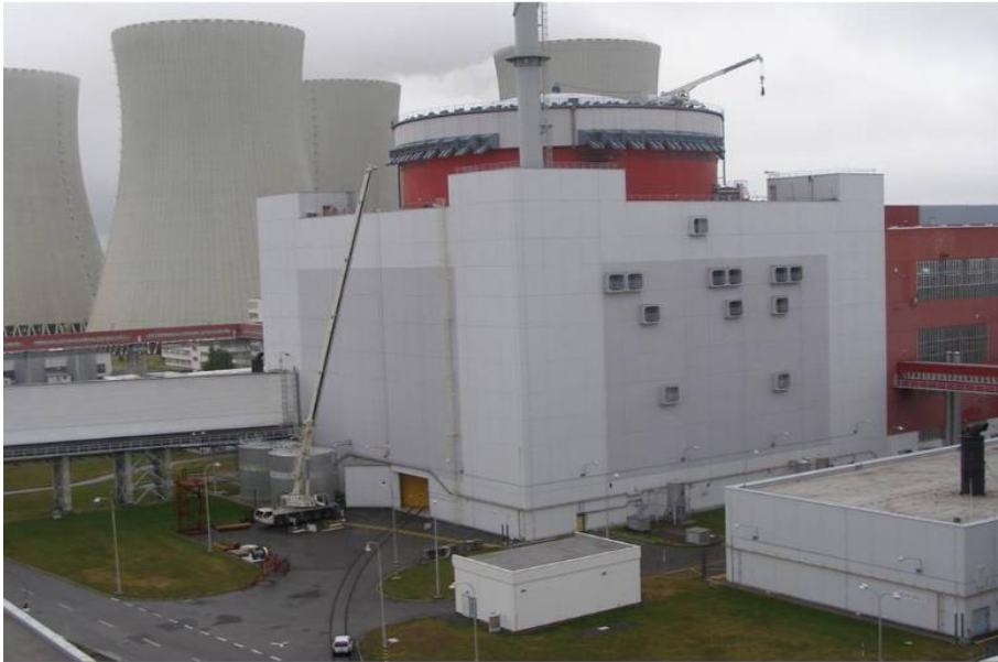
Photo of the containment surrounding building during the containment tendon maintenance
